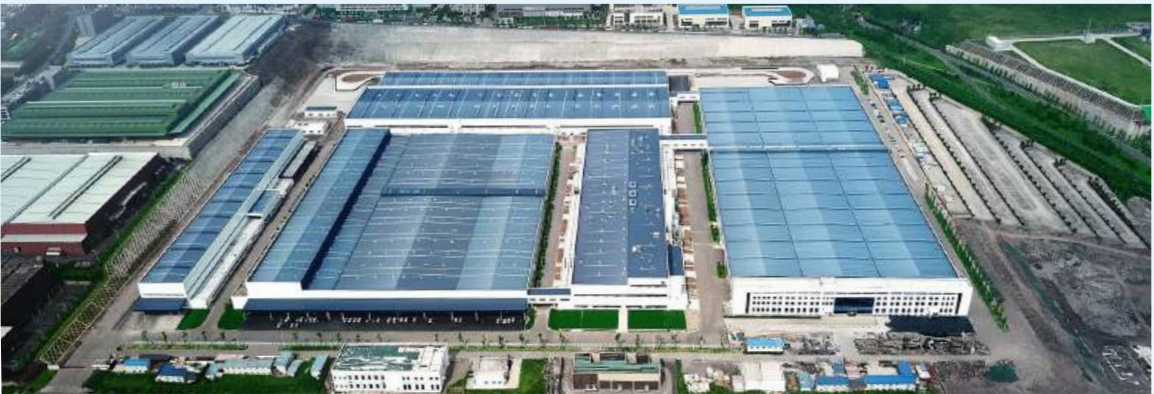
Intelligent Factory Photovoltaic Power Station
