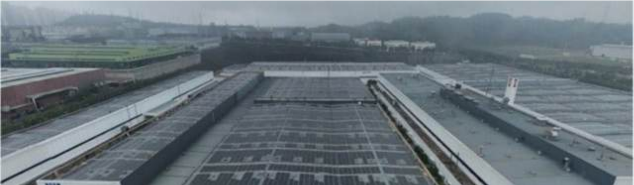
Solar photovoltaic power generation project
